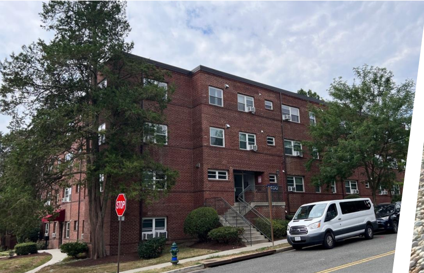
The red brick building post-rehab
