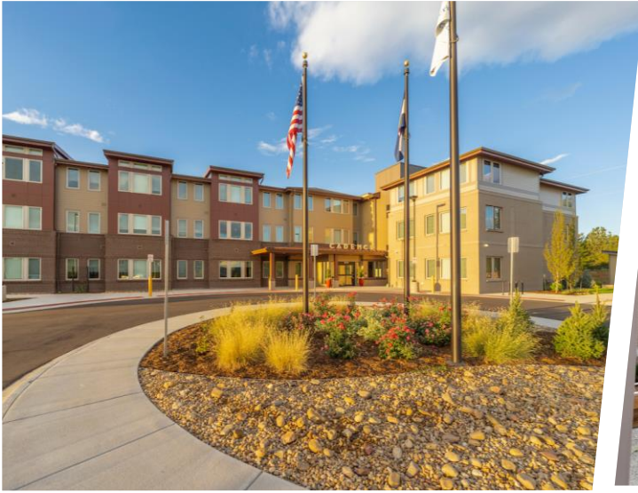
Cadence is the first new construction development to achieve Enterprise Green Communities Plus certification.
