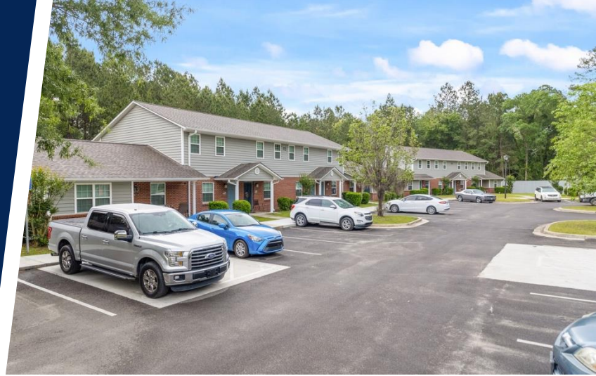
The Twin Oaks Apartments complex consists of seven buildings configured around a central community open space.
